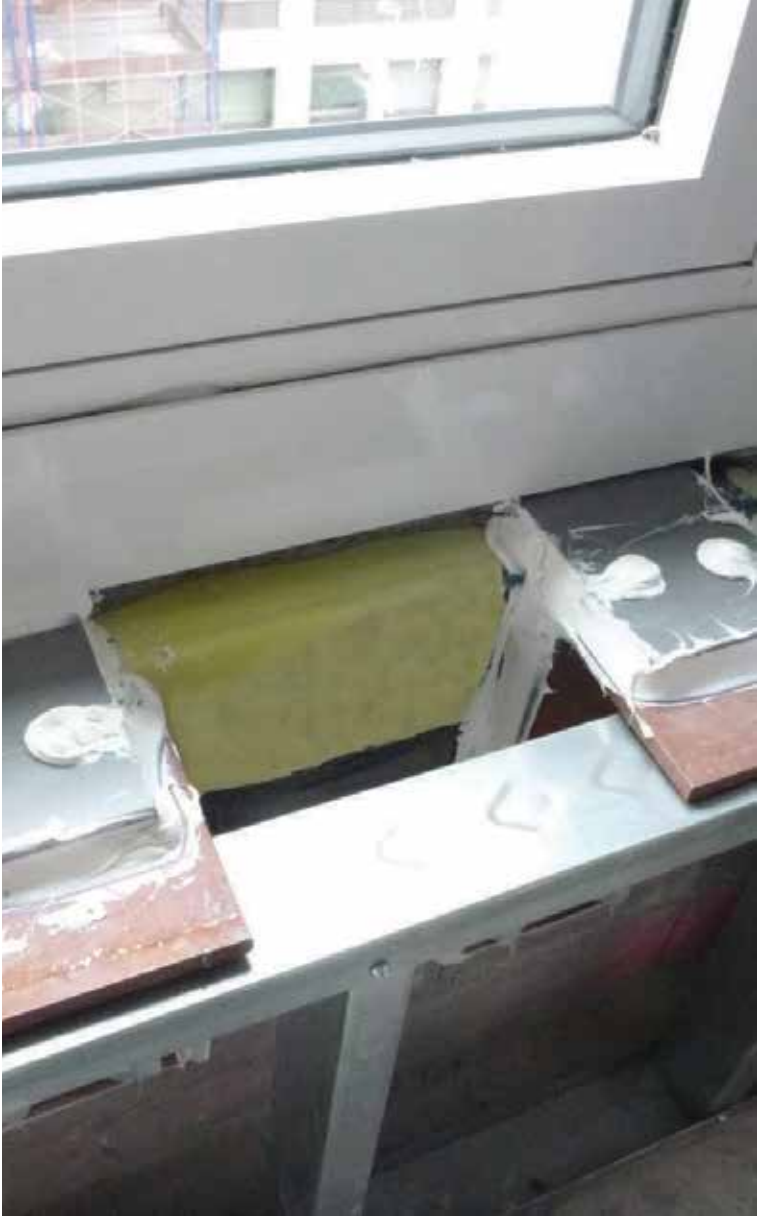
An example of high-efficiency detailing, where a thermal break is provided at point transmittances, such as metal-to-metal connections.
