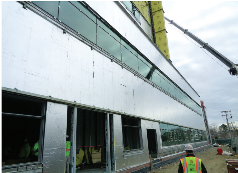
An aluminum-faced, impermeable air barrier with a rubberized asphalt adhesive applied to a fiberglass mat gypsum sheathing. The sealant is applied at several lap joints in the field of the air barrier installation to ensure continuity.
