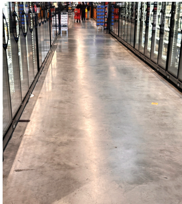
Despite this retail store being open for less than 18 months, the polished concrete finish has failed leaving an unsightly, pitted, unrefined concrete surface.
