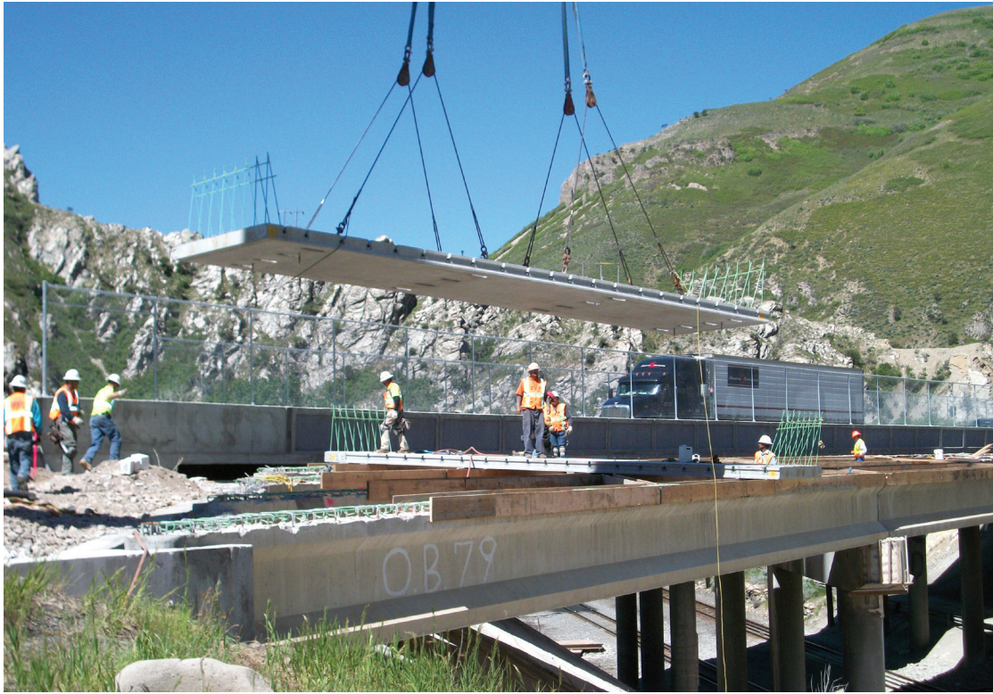
A pre-cast lightweight concrete bridge deck panel is carefully lifted into place as part of a resilient infrastructure project in a mountainous setting.
