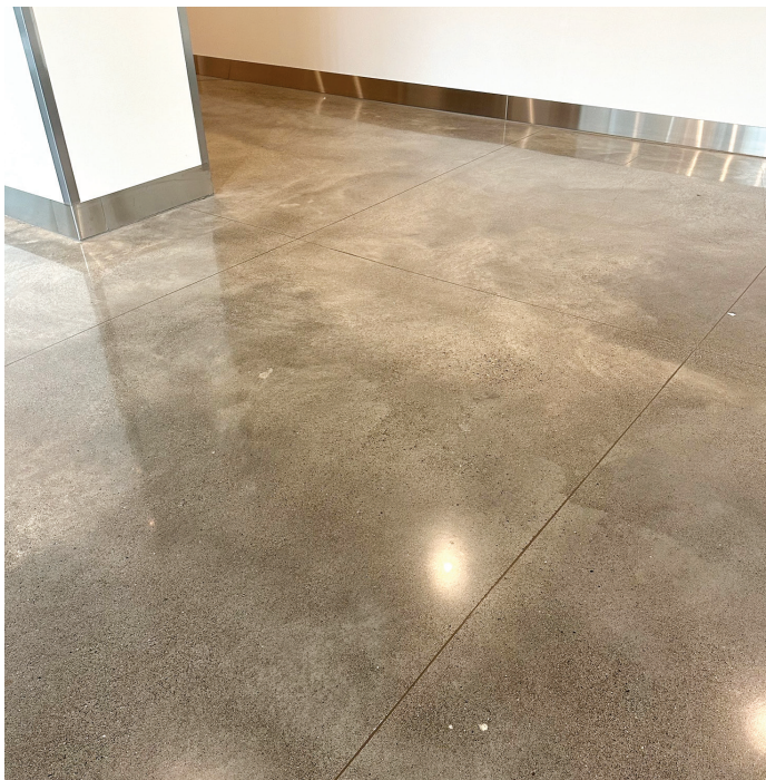
The refinement differences are clearly visible in this polished concrete image. It is likely that the benchmarks for this polishing scope were gloss-based and the design team had no way to protect the owner from this outcome.
