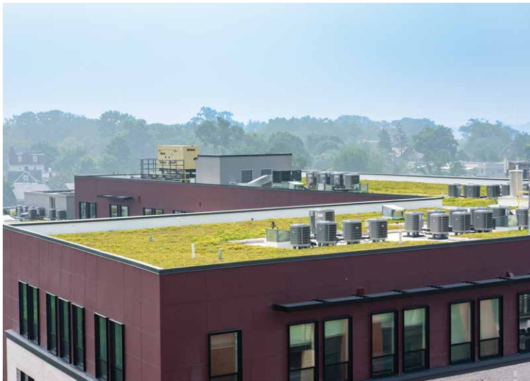
In total, the two facilities include 7,822 m 2 (84,200 sf) of roofing and approximately 4,775 m 2 (51,400 sf) of vegetative green roofing, which accounted for approximately 61 percent of the total roof area.
