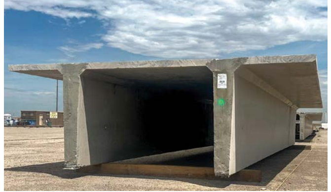
May precast concrete producers have invested in deep-stem double-tees to accommodate higher loads necessary for data center construction.
