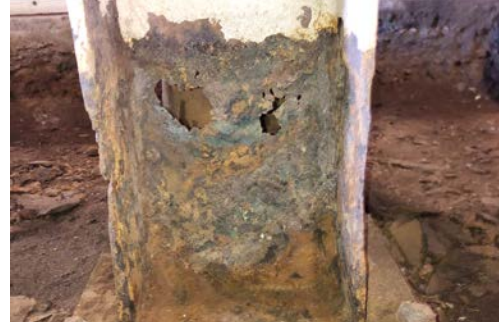
Corroded beam in sidewalk vault.
