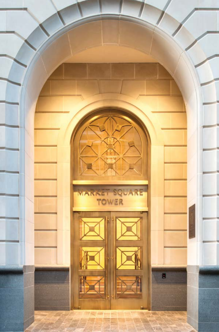
Bronze custom-balanced doors (formed bronze) installed at Market Square Tower in Houston, Tex.
