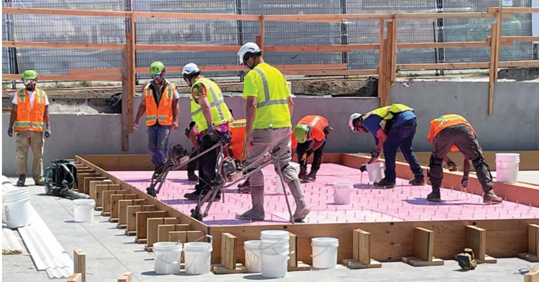
Teams anchor foam between panels after placing beauty panels.
