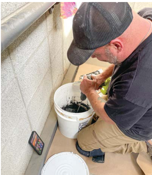
Thoroughly mix the epoxy, aggregate, and hardener.
