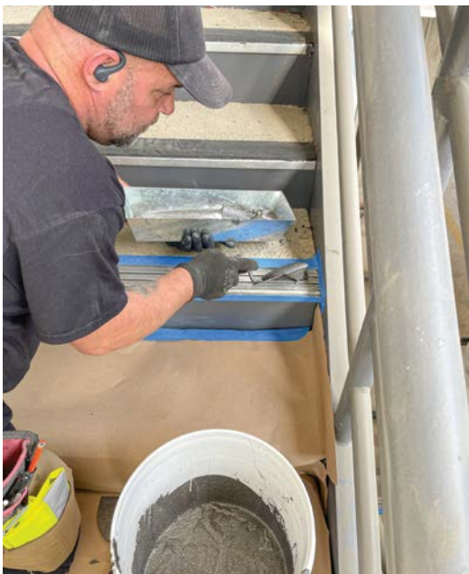
Applying thoroughly mixed DIY mixture to the prepared steps with a trowel or similar tool according to directions.
