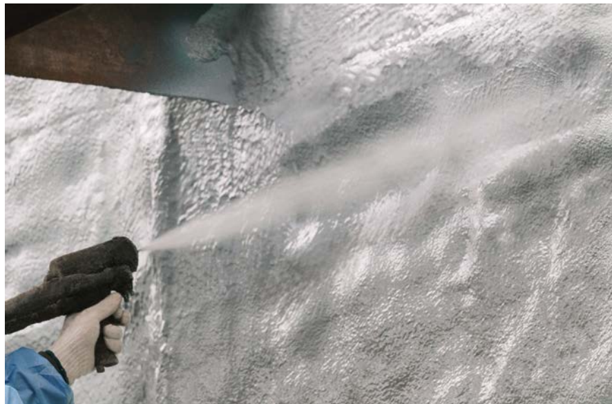
Contractor spraying the waterproofing coating over closed-cell sprayfoam.
