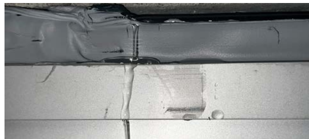
FIGURE 1: Close-up view of splice joint in metal sill trim that extends into the window rough opening, resulting in a discontinuity between the perimeter primary seal of the ribbon window system and the exterior wall assembly's water-resistive air barrier (WRAB).
