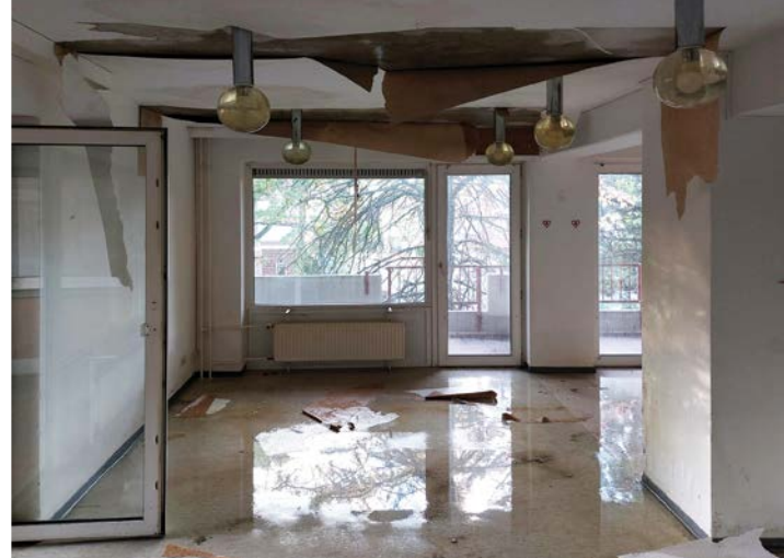
Interior flooding from 25.4 mm (1 in.) of water illustrates FEMA's estimate that even minor flooding can cause up to $25,000 in damage. Shallow water can compromise flooring, walls, and appliances, and lead to long-term health risks such as mold and poor indoor air quality.
