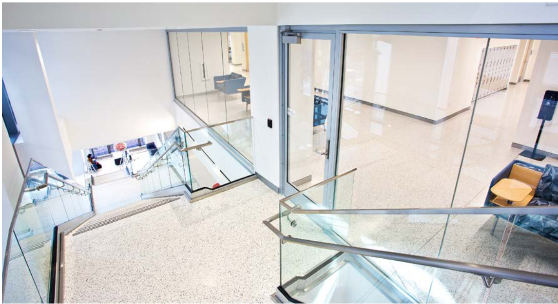
Minimal colorless spaces in these butt-glazed, fire-rated assemblies provide a cohesive design aesthetic with the stairwell's glass railings.
