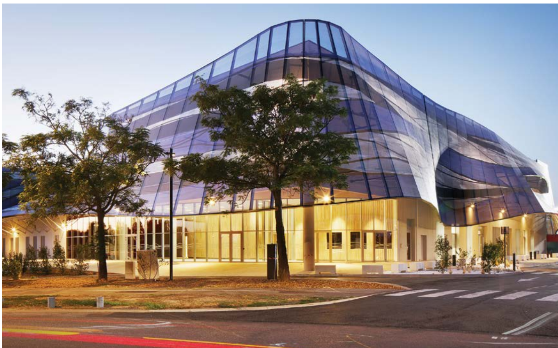
The Nîmes Sports Hall in France uses a 2,500-m 2 (26,909-sf) mesh designed for textile facades.
