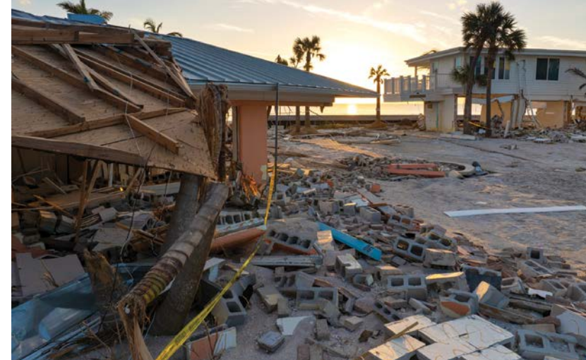
A beachfront home in Manasota Key, Fla., lies in ruins after Hurricane Milton's devastating impact. The storm's powerful winds and storm surge overwhelmed the building's defenses, leading to roof collapse and shattered windows. This destruction highlights the vulnerability of coastal structures to hurricanes and the importance of resilient building practices in these regions.
