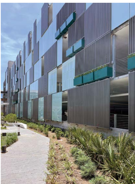
The parking facade project at the Mueller Parking Garage in Austin, uses more than 502 m 2 (5,400 sf) of laminated glass and louver panels.
