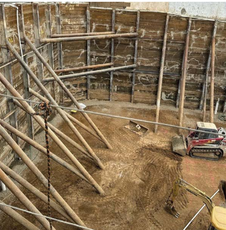
Back-lagged soldier pile lagging support of excavation with multiple bracing elements.
