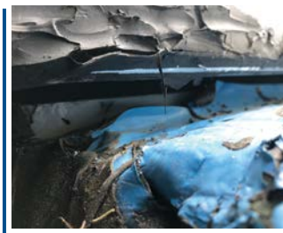
FIGURE 1: Close-up image illustrating poor quality of work and lack of proper integration between the unitized curtain wall and the field-installed accent panel assembly.
