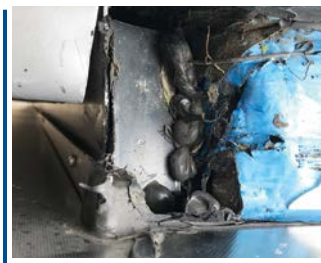
FIGURE 1: Close-up image illustrating poor quality of work and lack of proper integration between the unitized curtain wall and the field-installed accent panel assembly.
