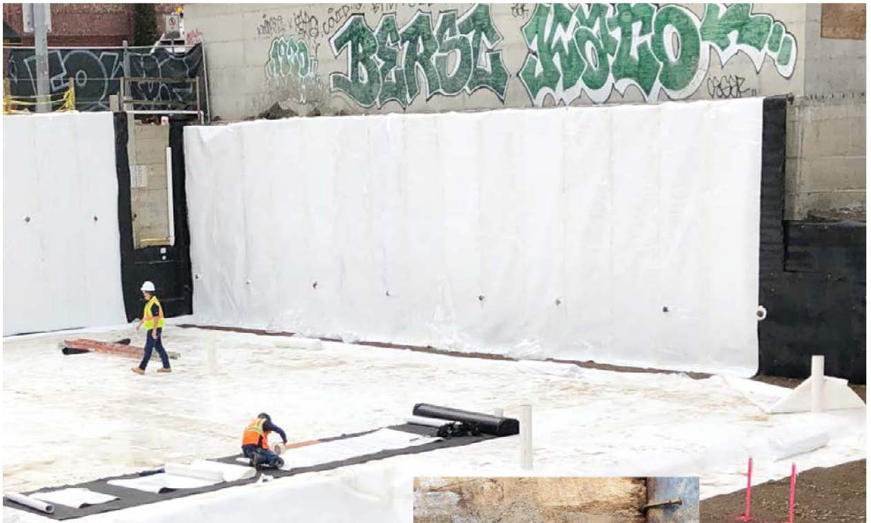
Above: First course of blindside waterproofing applied against soldier pile lagging.
