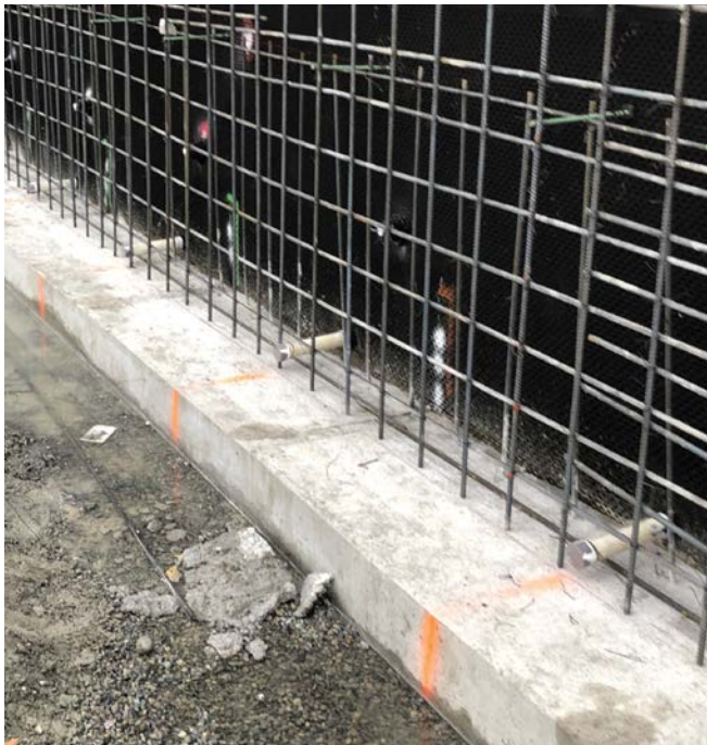
Drain outlets placed in the foundation wall to the interior subgrade of the structure.
