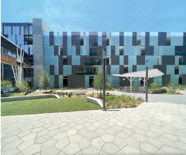
The parking facade project at the Mueller Parking Garage in Austin, uses more than 502 m 2 (5,400 sf) of laminated glass and louver panels.
