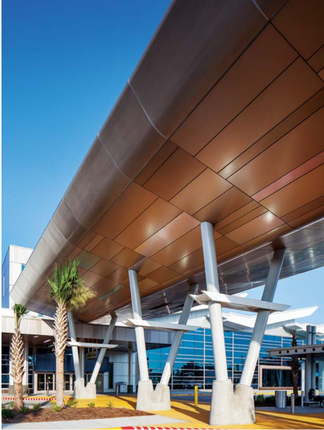
At Myrtle Beach International Airport, insulated metal panels (IMPs) in copper tones create a striking facade that elevates the architectural presence.
