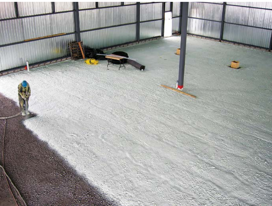
Open-cell spray foam insulation installed in a commercial building.
