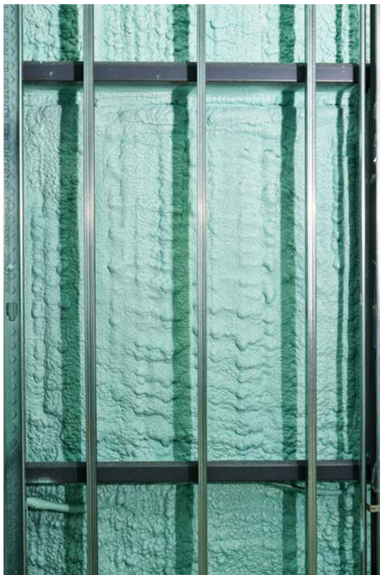
Closed-cell sprayfoam insulation applied in a metal construction building.
