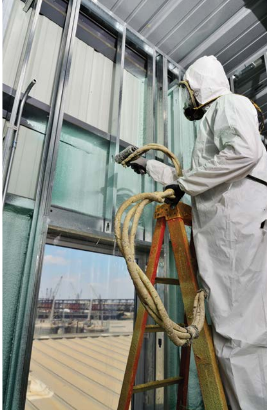
A professional sprayfoam contractor installing closed-cell sprayfoam insulation into a metal construction building.
