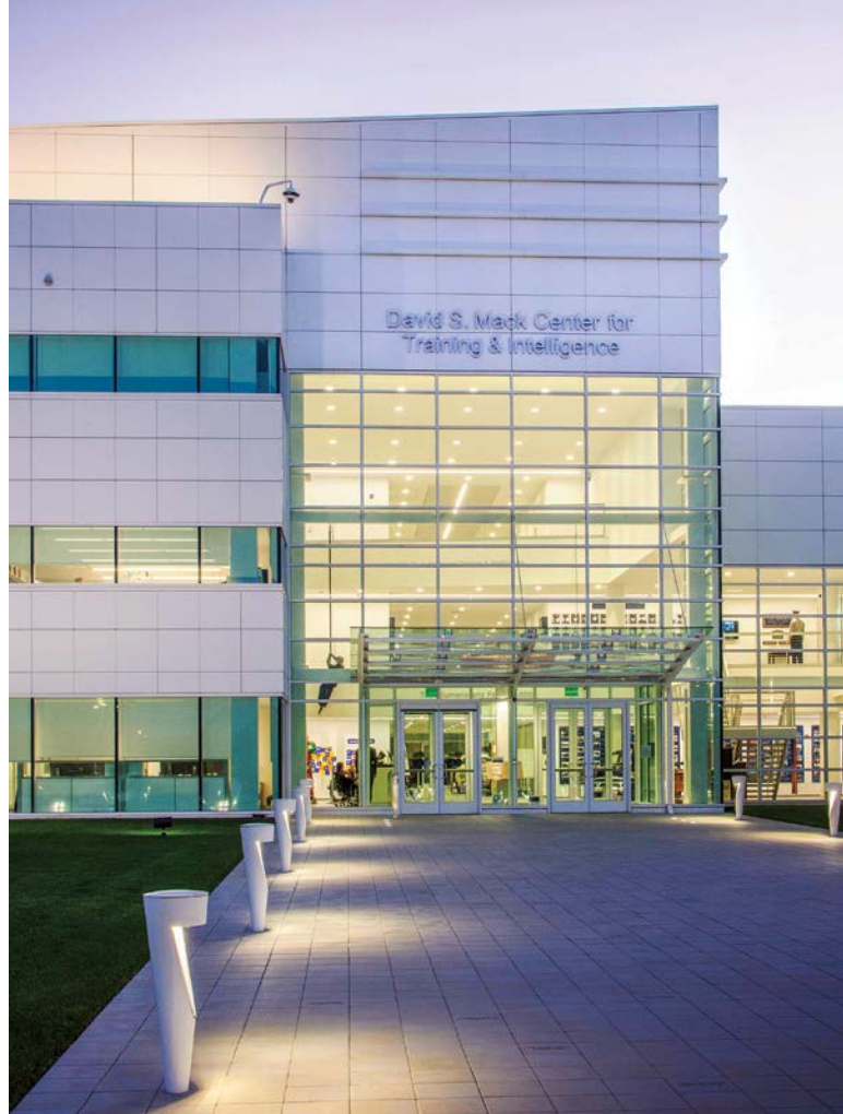
At the Nassau County Police Department, insulated metal panels (IMPs) and integrated design elements create a bold, modern civic presence.
