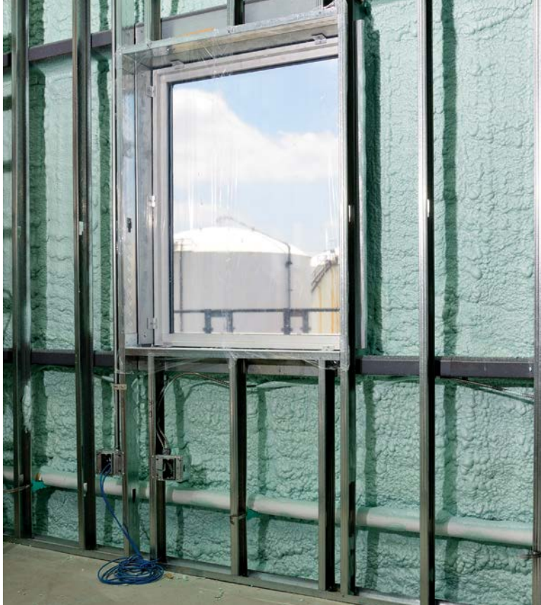
Closed-cell spray foam applied in a commercial building.
