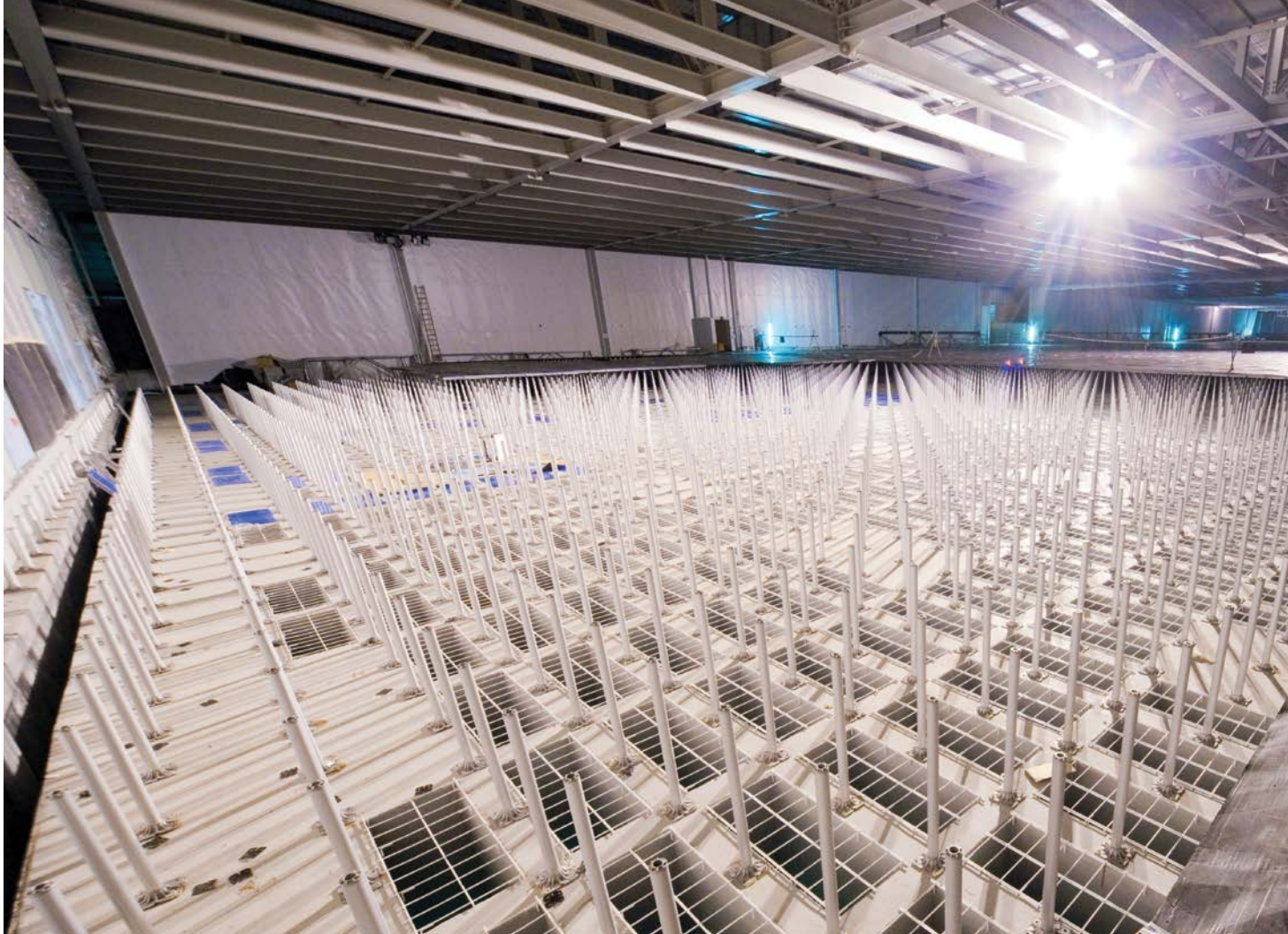
Interior view of waffle slab at semiconductor fabrication facility.
