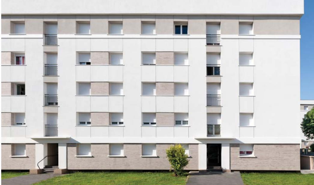
A thin brick cladding installed over continuous insulation (c.i.) in a rainscreen assembly, offering design flexibility without compromising energy efficiency.
