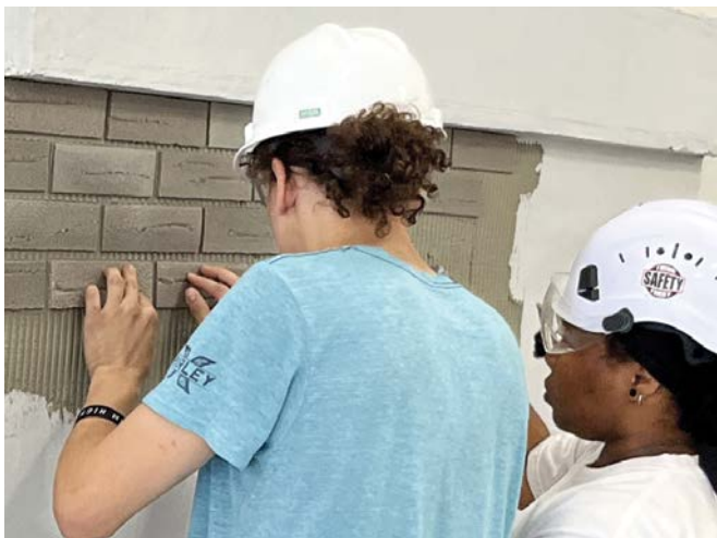
Field-application showing brick paneling, joint layout, and color range—an essential step for visual approval and quality control.
