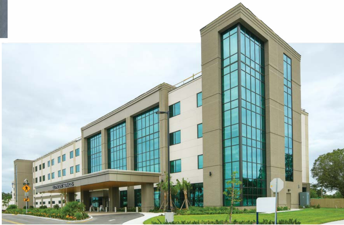
A lightweight, energy-efficient prefabricated exterior wall panels were used on this hospital expansion, combining the warmth of a brick aesthetic with faster installation, reduced on-site labor, and consistent quality control.
