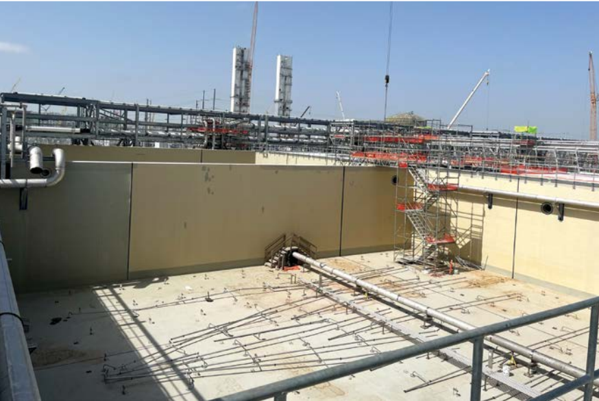
Steel framework of industrial water treatment under construction at a semiconductor fabrication plant.
