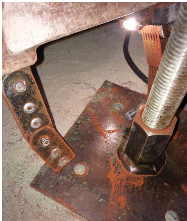
Magnetic particle inspection of welded joint.
