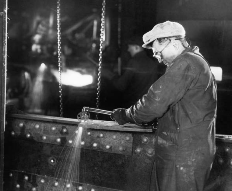
Early welding of structural steel.
