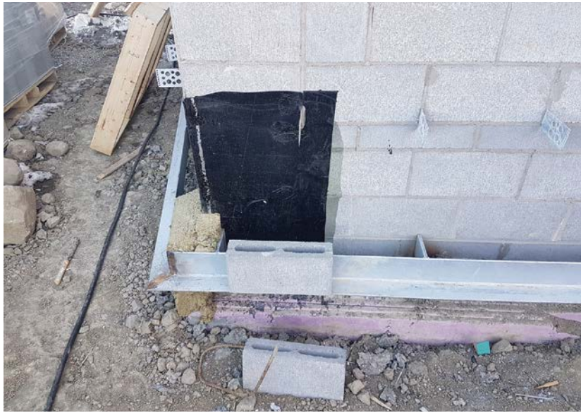
Knife plate standoff on a concrete block brick veneer wall assembly in a school.
