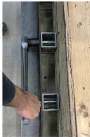
Knife plate standoff on a concrete block brick veneer wall assembly in a school.
