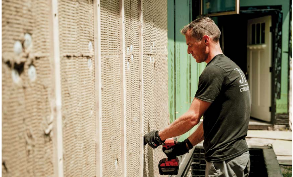
Installation of exterior noncombustible insulation.
