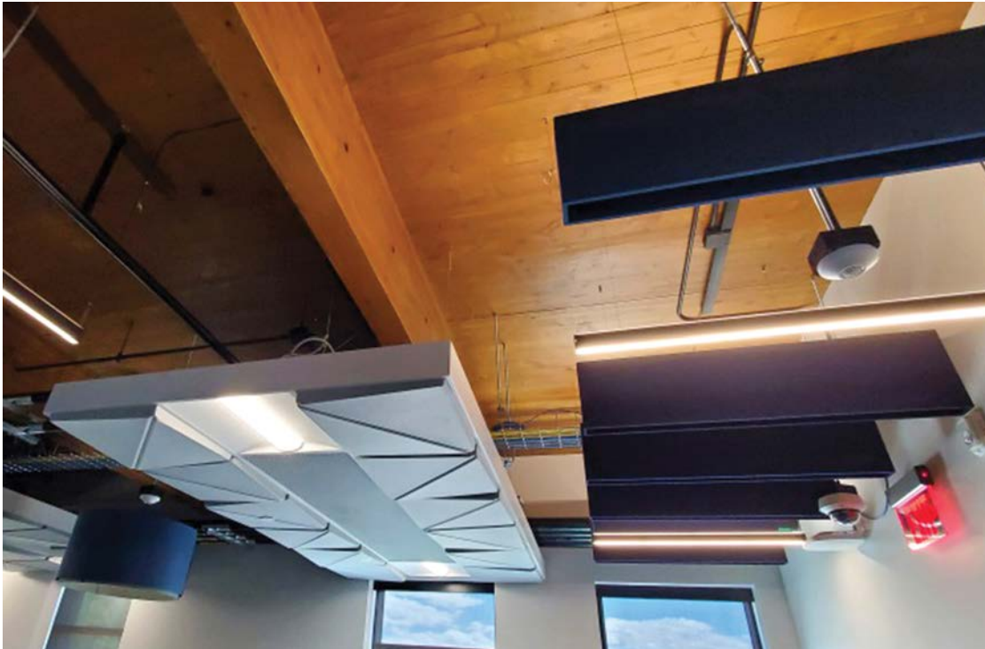
Mountain Line Downtown Connections Center's exposed chilled beams and acoustic treatments maintain optimal comfort levels.
