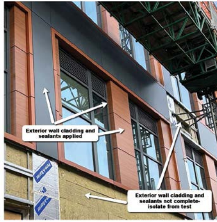
FIGURE 1: Exterior Wall Cladding and Associated Components Applied
