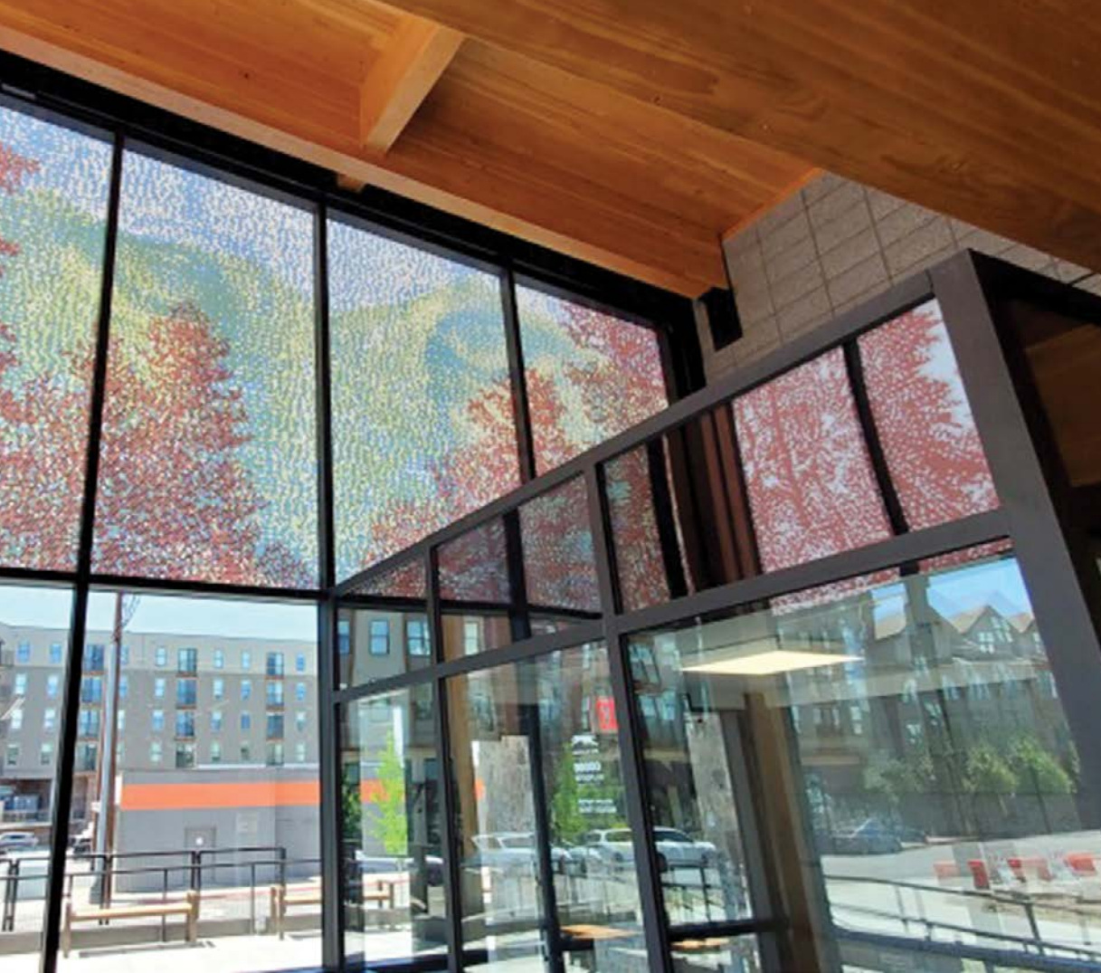
Mountain Line Downtown Connection Center's high-performance facade, enhanced by Haddad Drugan's artwork, Lion Eyes (Through the Forest) , allows the maximum potential for daylighting and a more engaging space.
