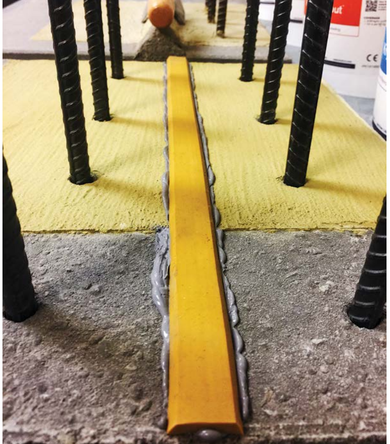
A swelling waterstop expands on contact with water to form a watertight seal at concrete joints, helping prevent infiltration over time.
