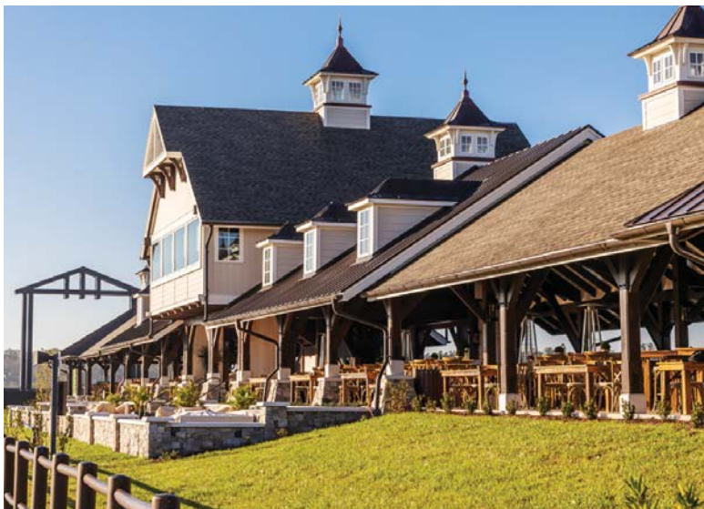
While Hurricane Ian destroyed other buildings in the area, TerraNova's viewing pavilion resisted the damaging winds and rain despite being directly in its path.
