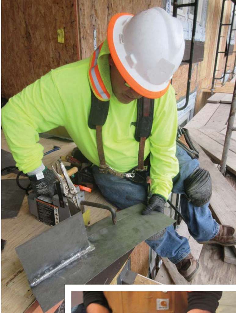
These photos illustrate the field fabrication, mechanical fastening, and soldering of galvanized sheet-metal flashing components and seams.
