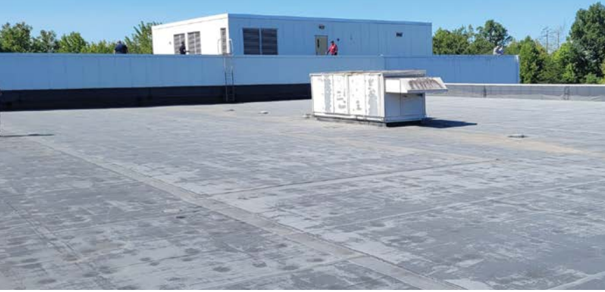
Existing low-slope roof conditions prior to restoration.
