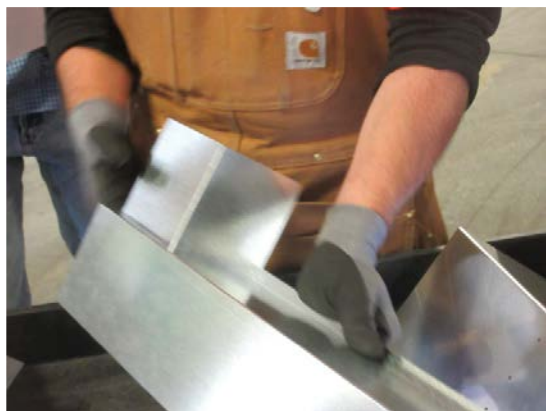
These photos illustrate the field fabrication, mechanical fastening, and soldering of galvanized sheet-metal flashing components and seams.
