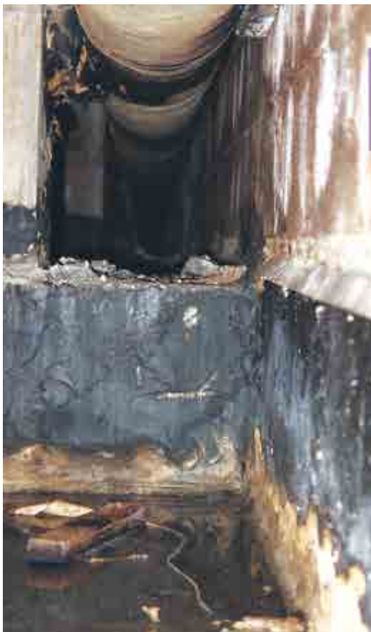
Deteriorated mortar joints on the outside wall pipe chase. (The access panels were built into the pipe chase structure.) The photo on the right shows inside the chase—note the the standing water at the bottom of the photo, along with the efflorescence on the exterior portion of the outside parapet wall.
