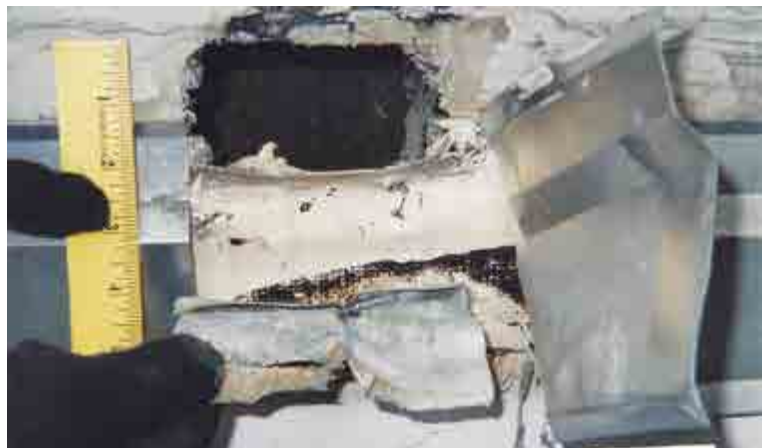
The two photos above provide close-up views of an improperly installed and deteriorated sheet metal through-wall flashing assembly. Inadequately installed sheet metal and surface-mounted counterflashing can be seen.
