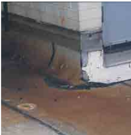
Southeast corner of the mechanical room elevation structure. Note the dissimilar materials added to the bottom and the surface-mounted counterflashing at the base of the door threshold. In the close-up at right, the counterflashing has been taken apart; the original sheet metal through-wall flashing is buried in the wall behind the new base flashing material.
