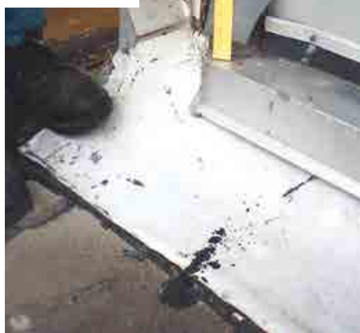
Southeast corner of the mechanical room elevation structure. Note the dissimilar materials added to the bottom and the surface-mounted counterflashing at the base of the door threshold. In the close-up at right, the counterflashing has been taken apart; the original sheet metal through-wall flashing is buried in the wall behind the new base flashing material.
