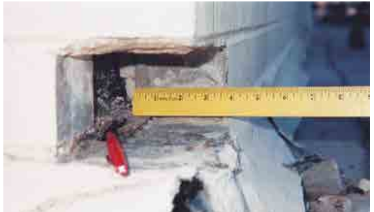
In this project, lifting back the improperly installed sheet metal counterflashing reveals the height of the base flashings are improperly installed and terminated less than 200 mm (4 in.) higher than the finished roof surface.
