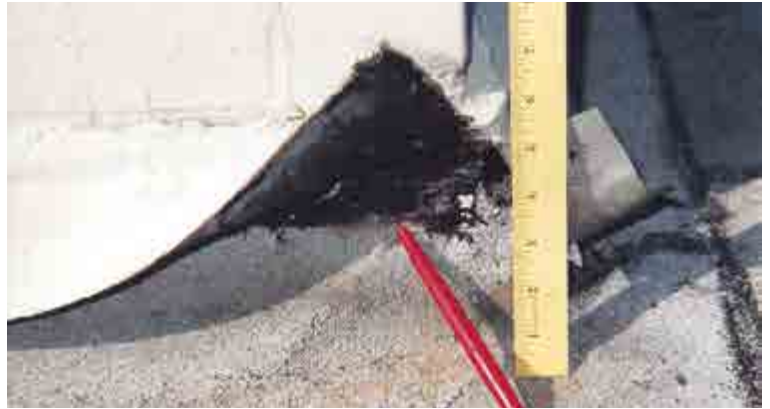
In this project, lifting back the improperly installed sheet metal counterflashing reveals the height of the base flashings are improperly installed and terminated less than 200 mm (4 in.) higher than the finished roof surface.
