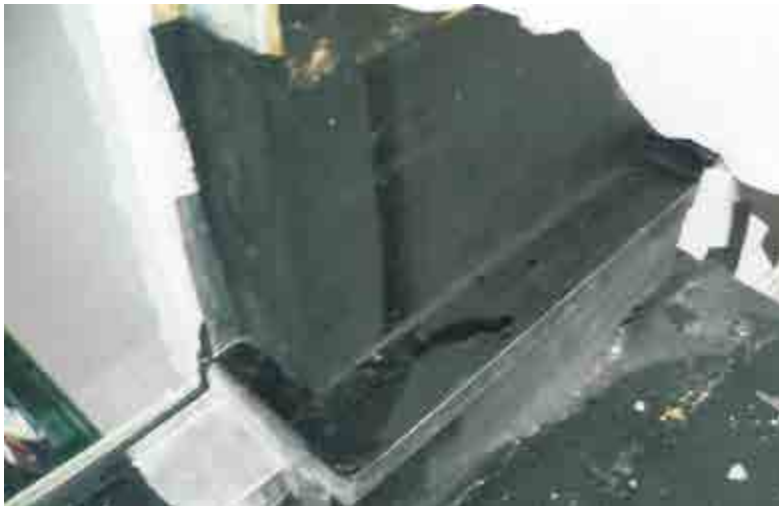
A close-up view of a properly installed through-wall flashing assembly. There is lead-coated copper sheet metal flashing covering over, and soldered above, a field condition at the left-hand portion of the assembly. Additionally, note the end dam at the upper right-hand portion of the photograph.
