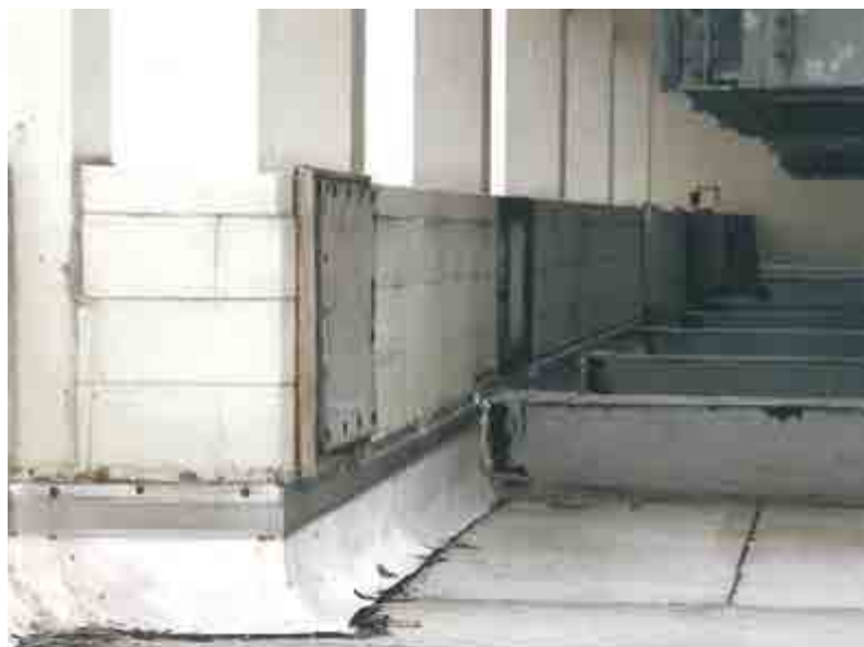
Deteriorated mortar joints on the outside wall pipe chase. (The access panels were built into the pipe chase structure.) The photo on the right shows inside the chase—note the the standing water at the bottom of the photo, along with the efflorescence on the exterior portion of the outside parapet wall.
